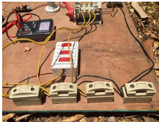
Figure 5: Measurement of Grid connection
