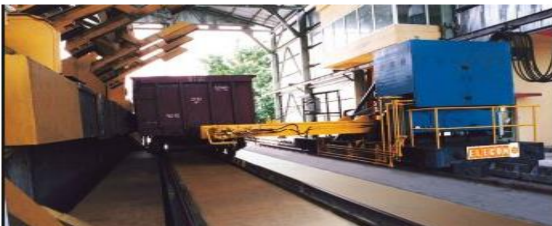
Figure 1.3: A snap shot of Side Arm Charger positioning the wagon in Tippler area
